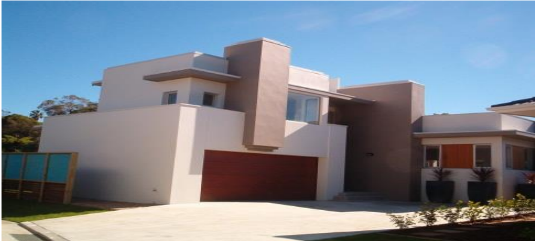
Figure 11: Exterior of a house with external walls made of concrete blocks. Photo by
